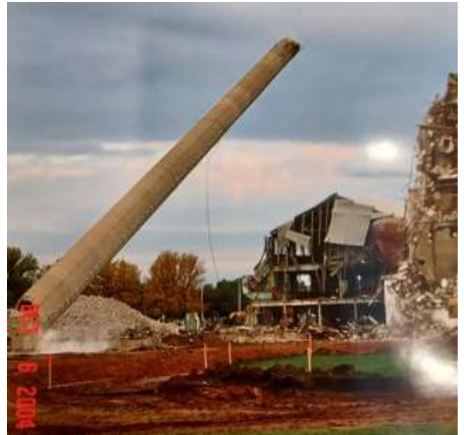
Smoke stack coming down in 2004
